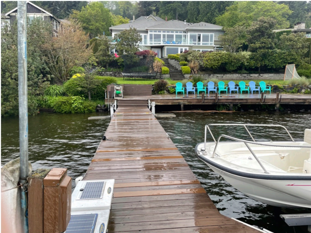
Photo 2 - Existing dock looking landward.
