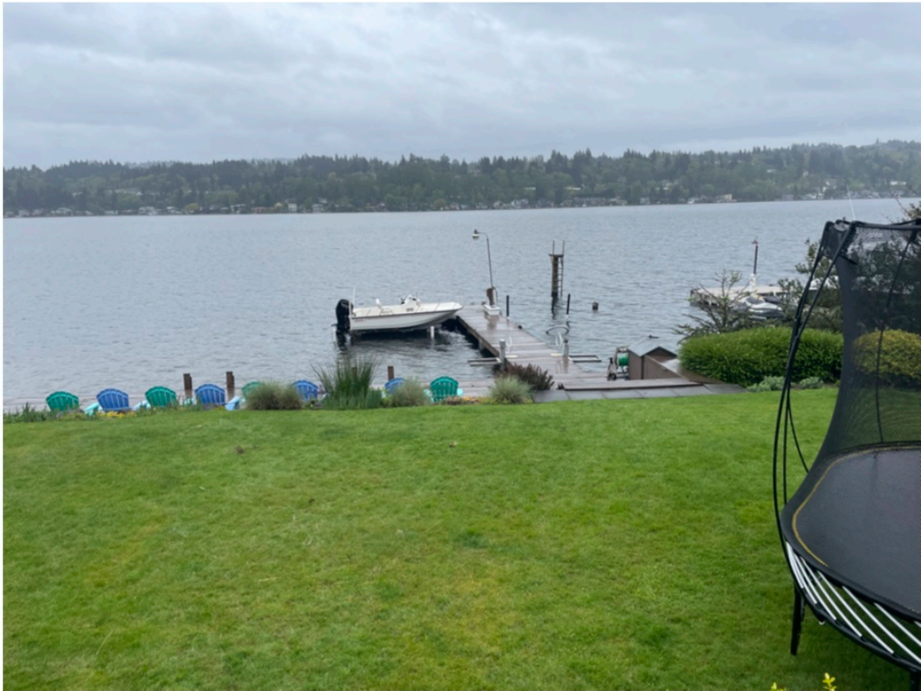
Photo 1 - Existing dock looking waterward.
