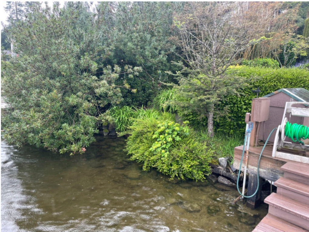
Photo 4 - Shoreline conditions south of the dock.
